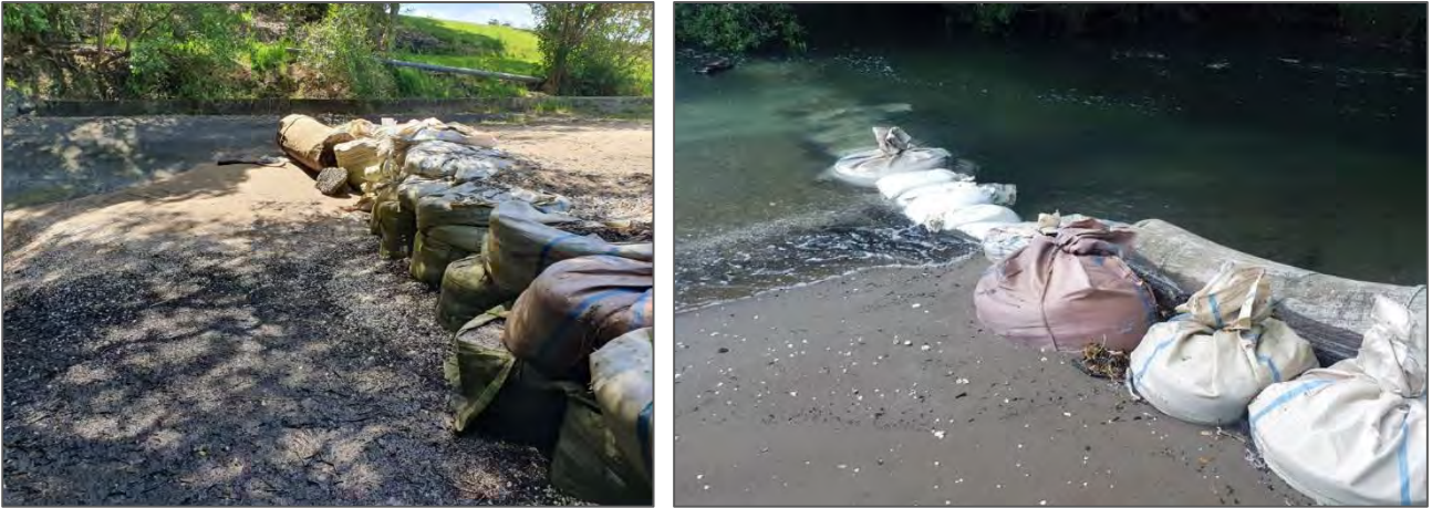
Figure 14. Groyne structure consisting of commercial sandbags with the aim of disrupting the cross-shore sediment movement (Left: Photograph from WSP site visit on the 30 th of October 2019; Right: Stuff.co.nz (July 31 st 2019).
