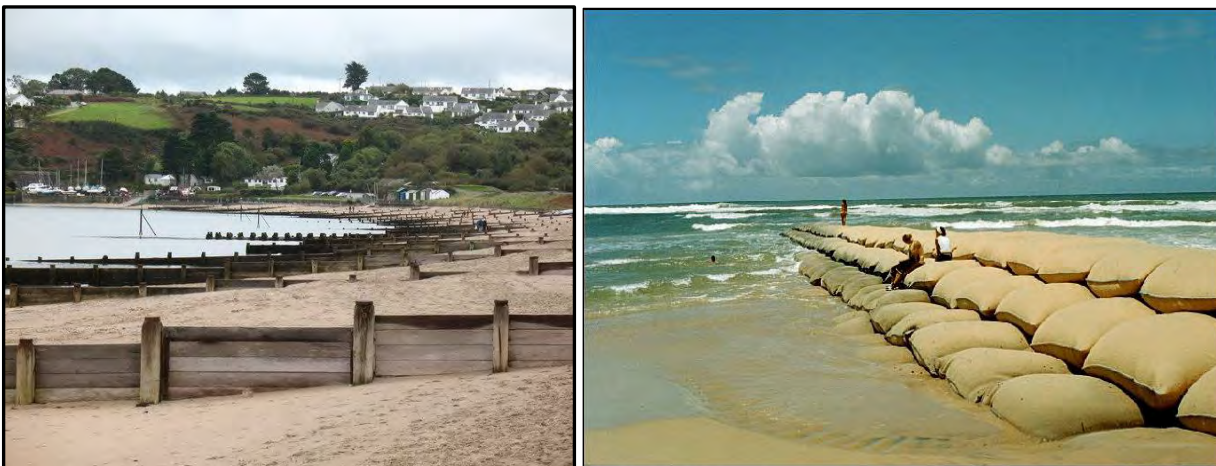
Figure 24. Timber and geotextile sand filled containers. (Photographs sourced from geograph.co.uk and researchgate.net respectively. Last accessed 22 nd November 2019). Note these structures may not be appropriate for Little Shoal Bay
