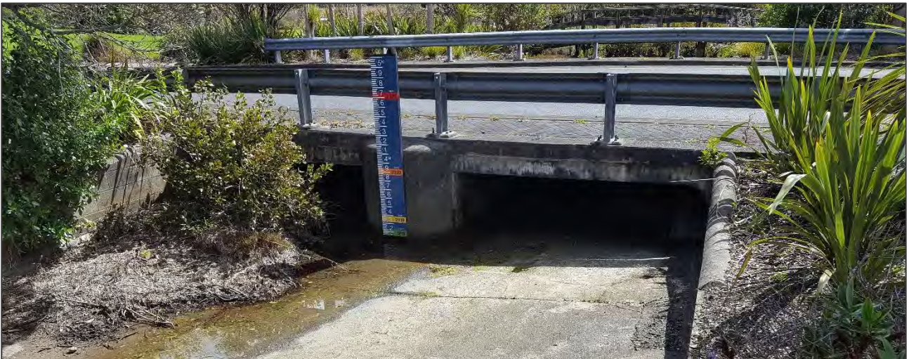
Figure 18. Box Culverts in Little Shoal Bay, showing the left box culvert partially blocked by debris and vegetation
