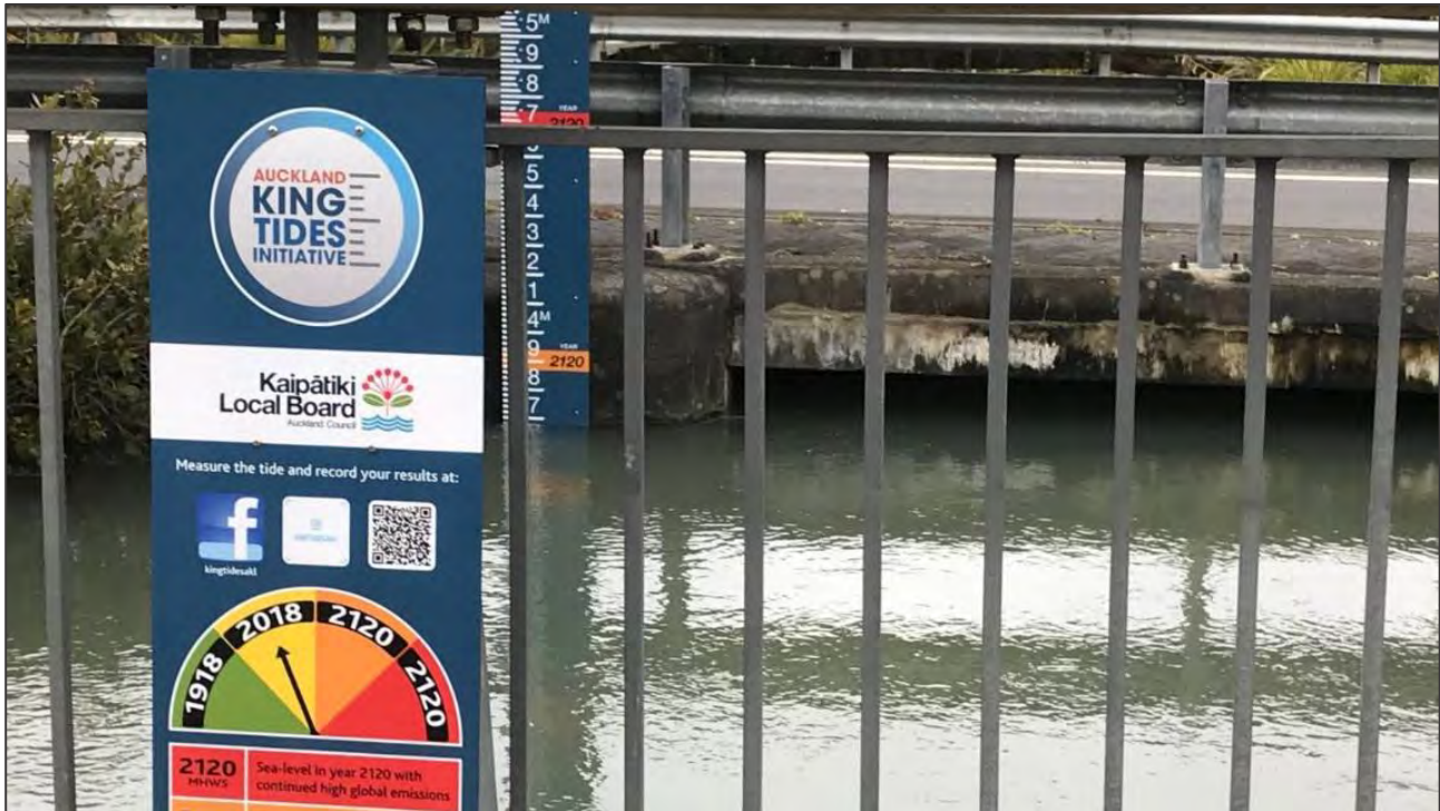
Figure 23 - Box Culverts in Little Shoal Bay, showing a mean high springs scenario almost reaching the orange line, which represents a water elevation prediction as best-case scenario of greenhouse gas emission until 2120 (Source: Stuff - Little Shoal Bay: Rising sea level)
