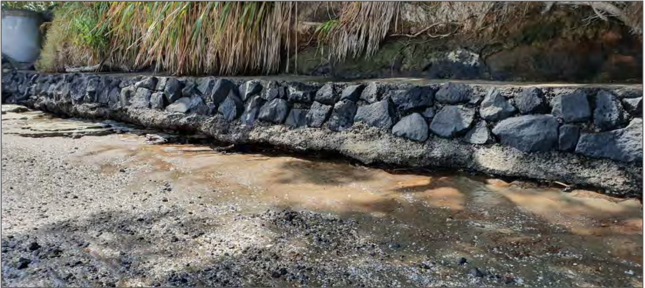
Figure 9. Undermining of gouted rock seawall on the eastern boundary of Little Shoal Bay.
