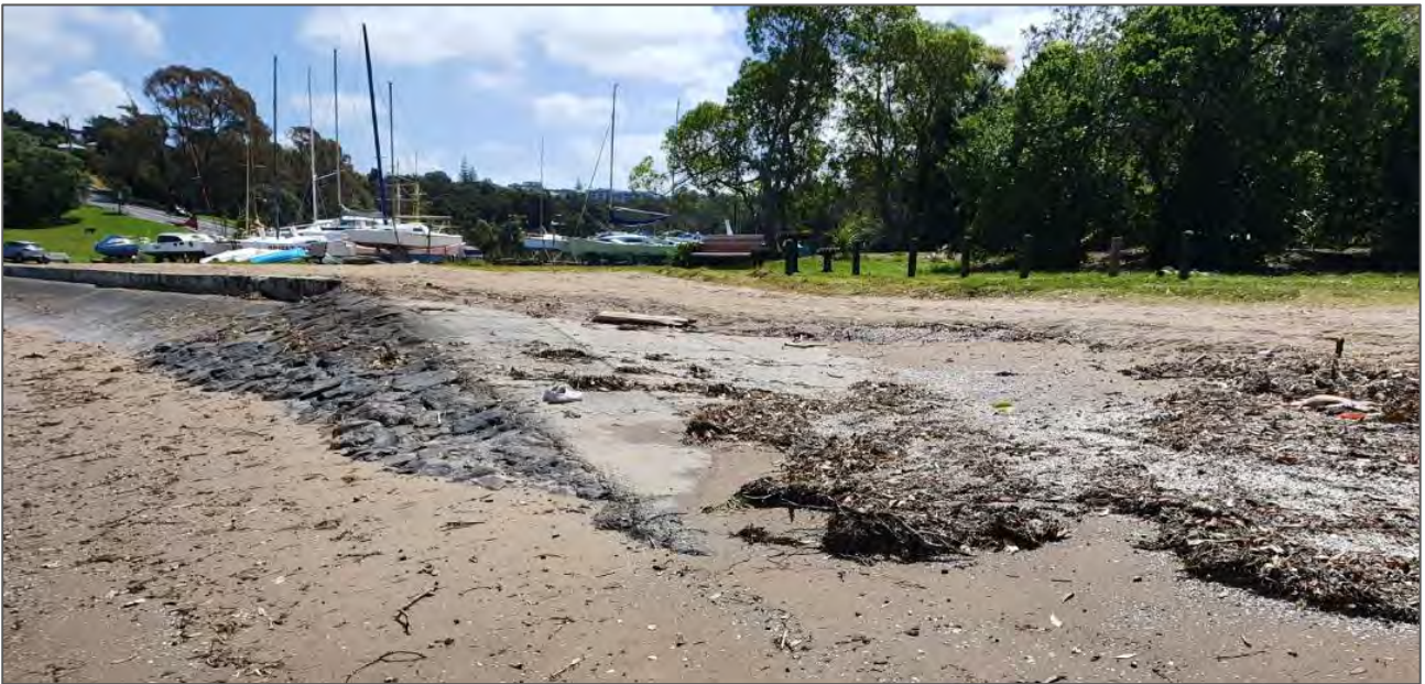
Figure 16. Debris and sediment accumulated on the top of the boat ramp
