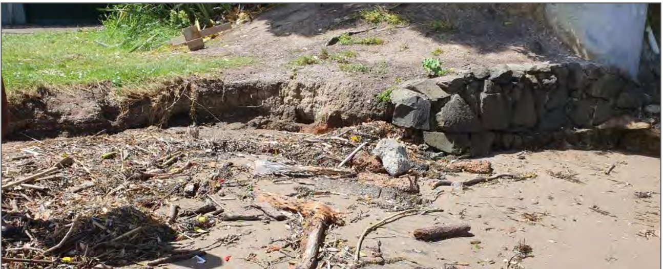
Figure 10. Localised erosion on the eastern side of bay
