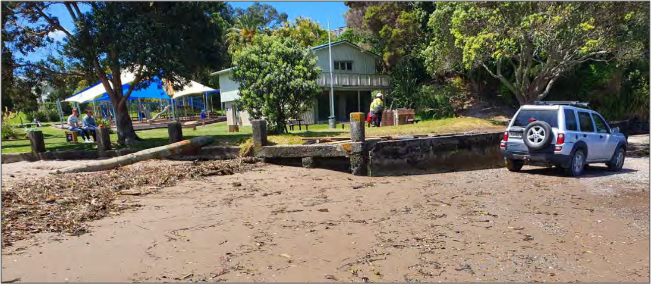
Figure 11. Eastern side of Little Shoal Bay showing accumulation of sediment and debris.
