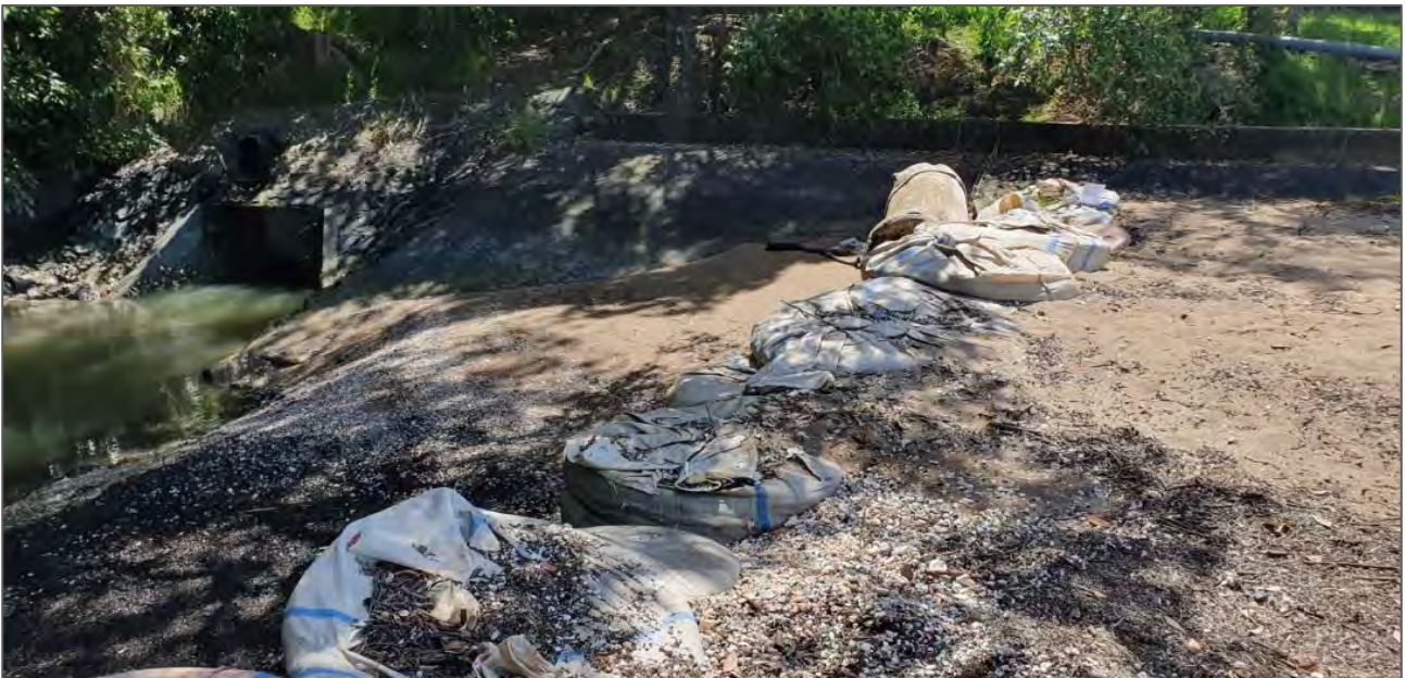
Figure 13. Construction of groyne structure to retain sediment on the eastern side, and the outlet located on the west of Little Shoal Bay
